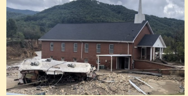
Flooded church and RV near I-26 in Erwin/Unicoi County.
