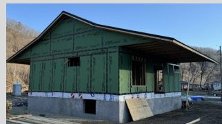
House #1 under roof
