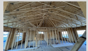
Inside progress as of 1/9
